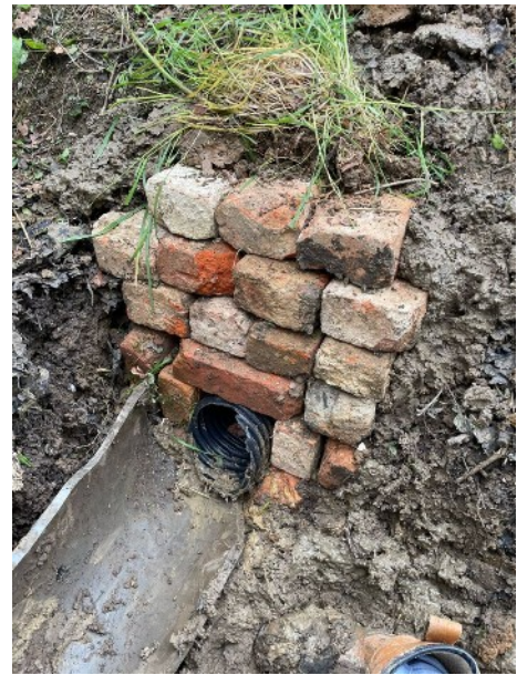
the drainage pipe outlet
