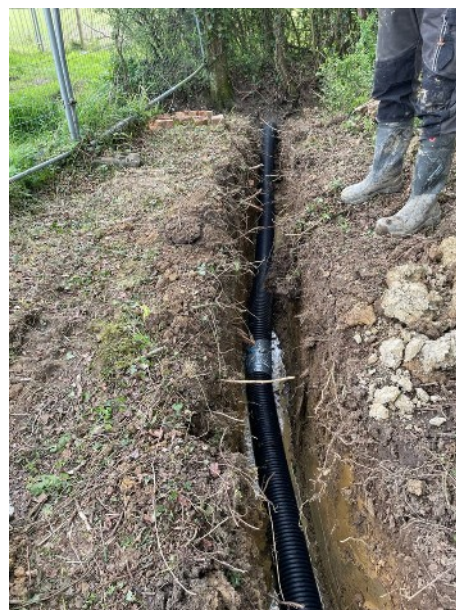
the new drainage ditch and pipe
