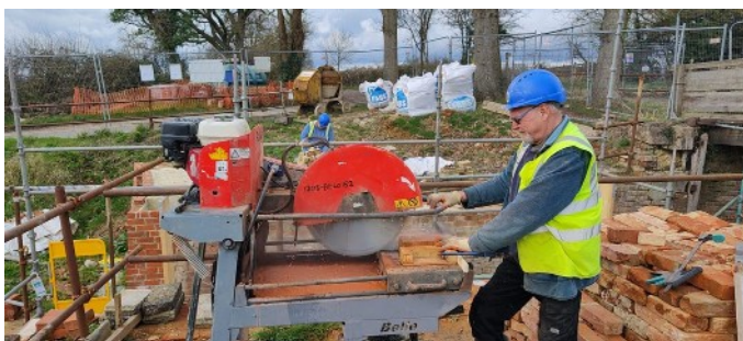
Roger lining up the brick cutter prior to operation
